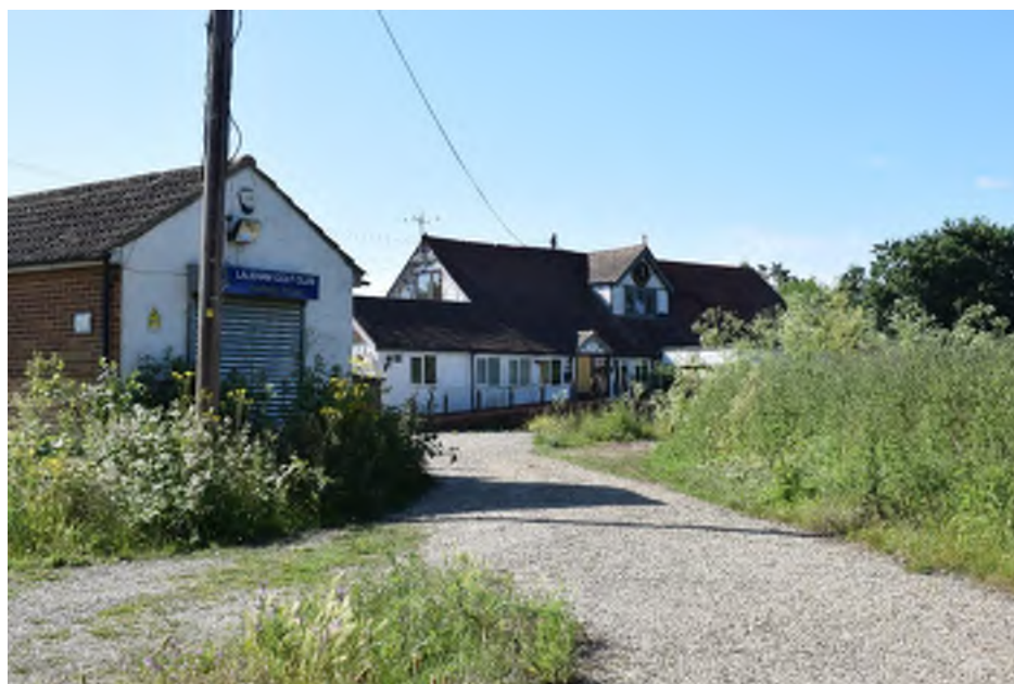
Plate 16: Views south to the former Laleham golf club building situated on the north bank of Thames Side. Grounds are overgrown and fenced off from public access.
