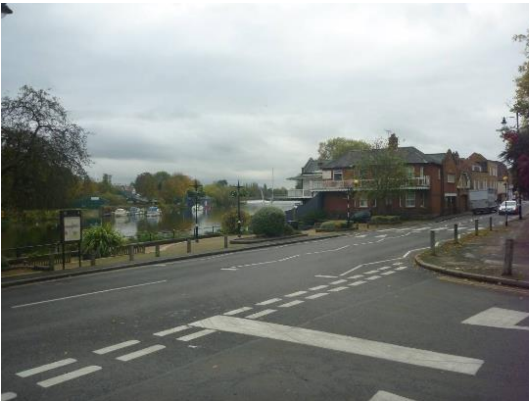
View of Sunbury Weir from the edge of the Lower Sunbury Conservation Area
