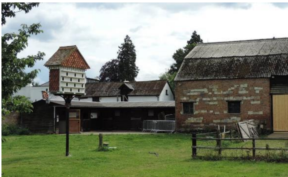
172 Dovecote in Farmyard of Abbey Bridge Farm
