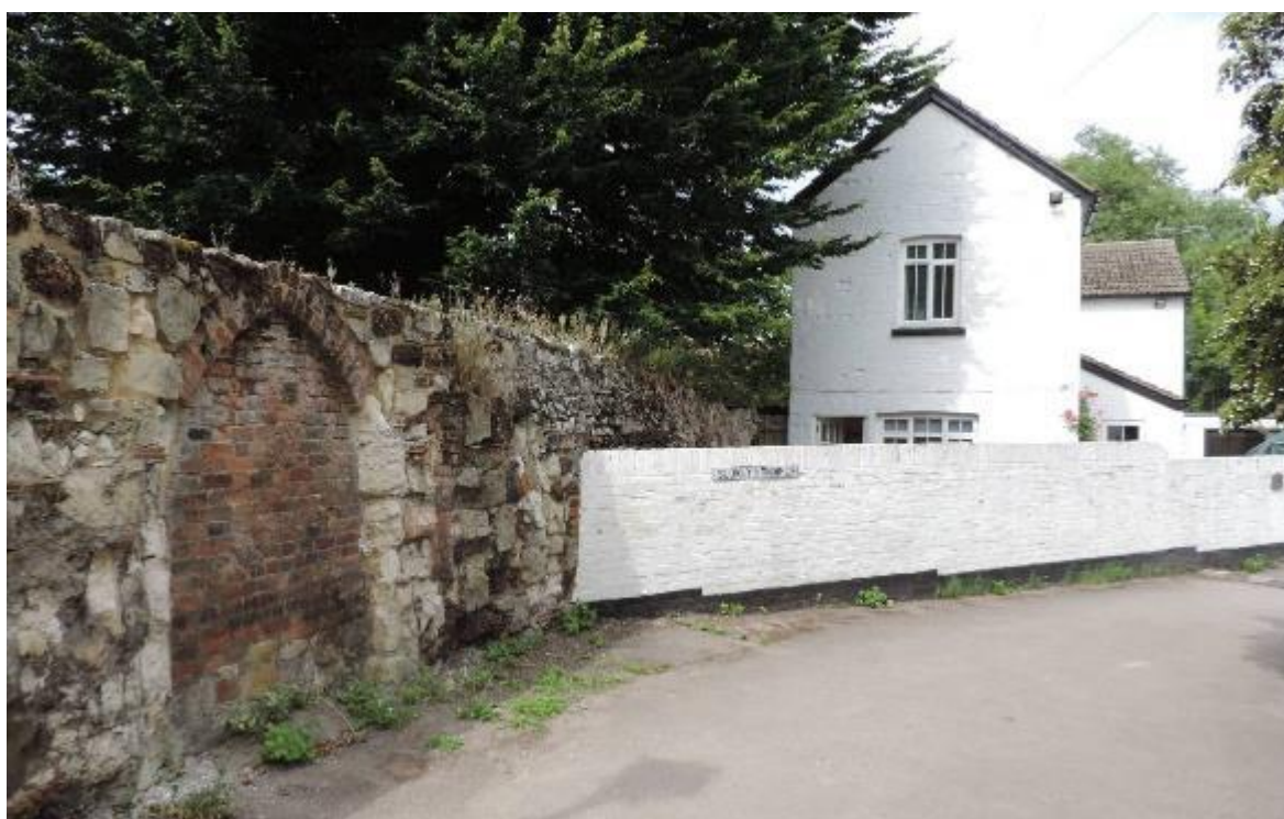
163 Medieval doorway in garden wall of Abbey House
