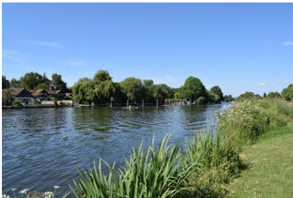
Plate 24: Approximate location of the proposed Sunbury Weir fish pass, views looking north-east across the existing Weir.
